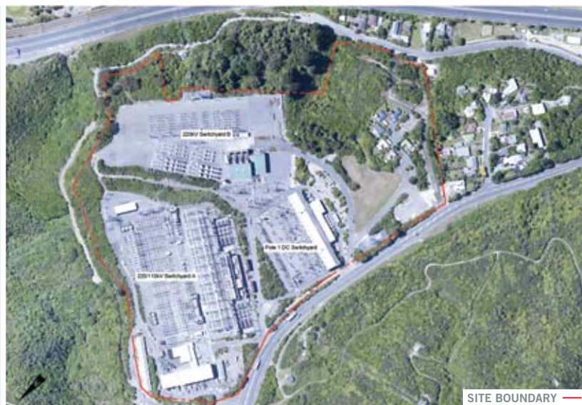
Existing Haywards → substation
