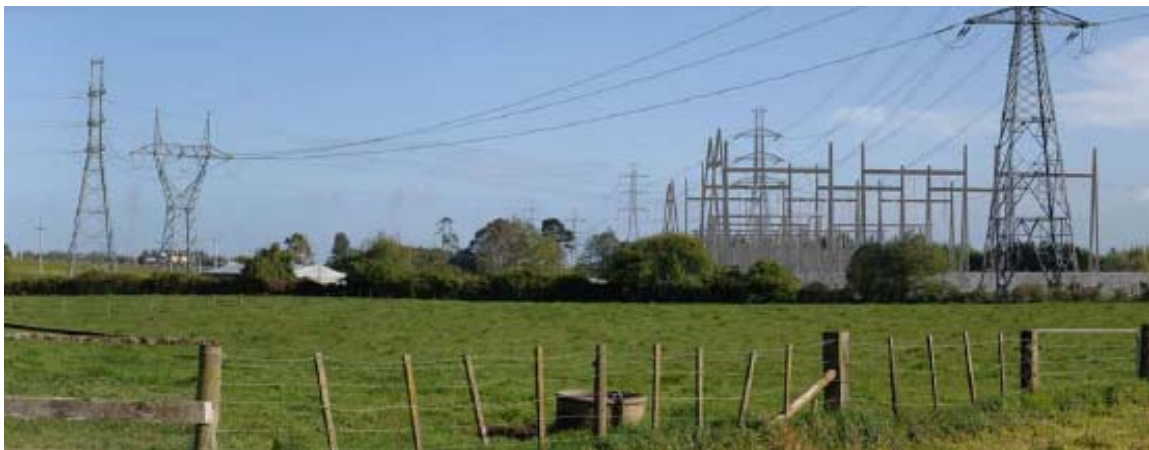
Figure 3: Simulation of the Drury Switching Station – Our First IEC 61850 Deployment
