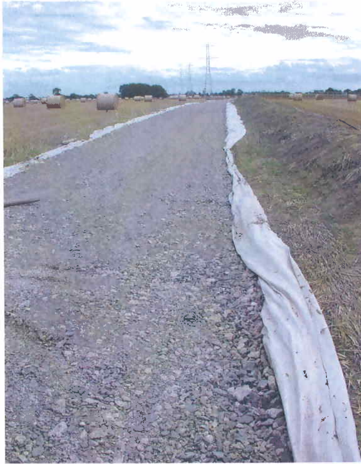
Image 1: Road construction using Geotextile
