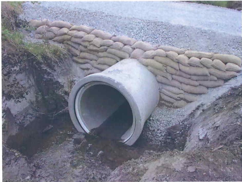
Image 2: Culvert installed in drain crossing
